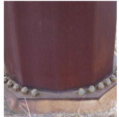
Weathering steel electrical distribution pole
