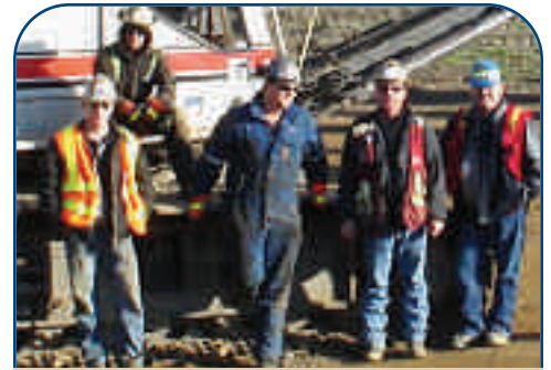
NORTH AMERICAN CAISSON LTD. VOYAGEUR DRIVING PILES AT VOYAGEUR
