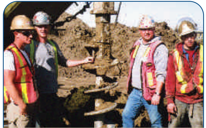
NORTH AMERICAN CAISSON LTD. - CODA ATHLETIC AND ICE COMPLEX CANADA OLYMPIC PARK MEMBERS WORKING ON THE FUTURE HOME OF HOCKEY CANADA
